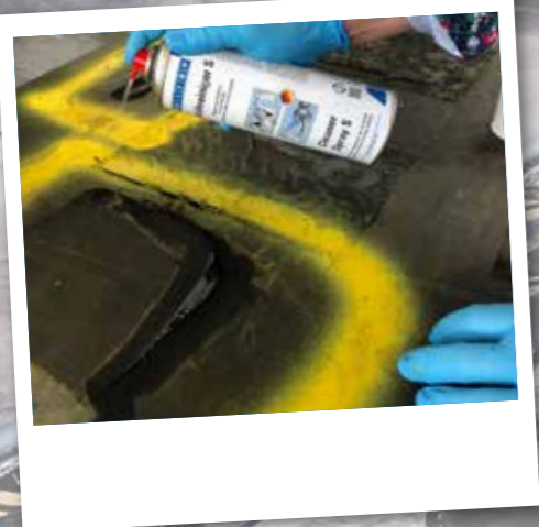
First, the conveyor belt was cleaned with WEICON Cleaner Spray S.
