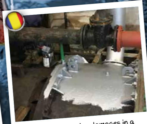
Repair of corrosion damages in a hydroelectric power plant
