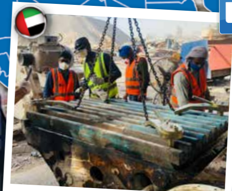
Gap filling on a press plate
