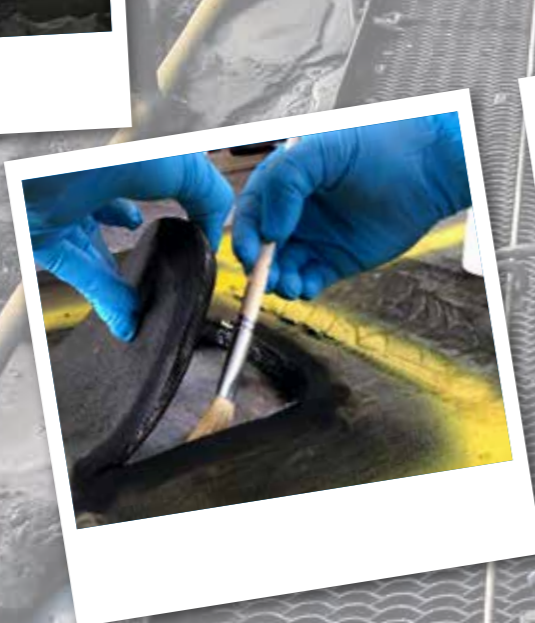
Then, WEICON Primer G was applied. The bonding agent ensures a better adhesive joint for surfaces that are difficult to bond - like rubber, in this case. That way, the adhesive bonding was ideally prepared. Then, the WEICON Urethane 85, which is included in the WEICON Belt Repair-Kit, was worked in and moulded to match the surface of the conveyor belt.
