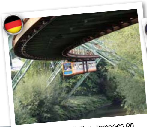
Repair of cavitation damages on bridge girders
